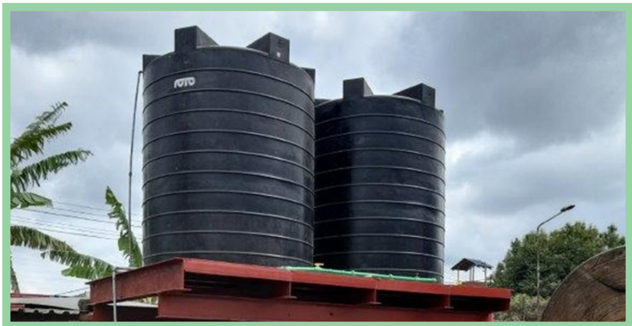
Constructed a water tower
