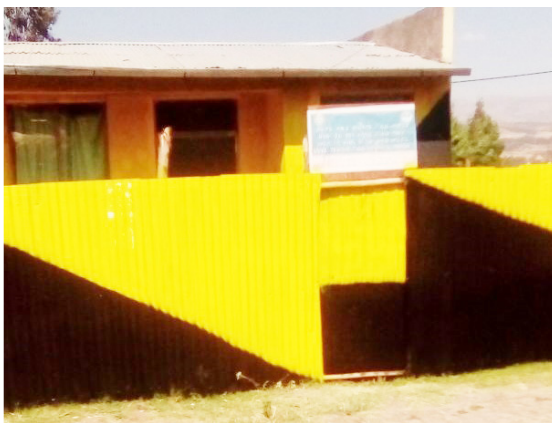
▶ Roto Ethiopia renovated the community police station
