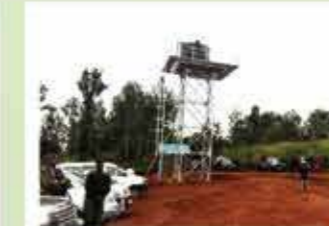
Gathuri Community Water Project
