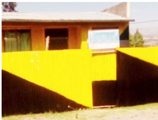
▶ Roto Ethiopia renovated the community police station
